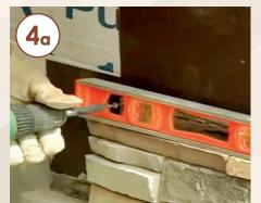
The most important part of the entire installation process is getting this first course of stone perfectly level. It will act as a foundation for the rest of the wall and makes for a smoother and more secure process.
