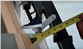
Moving steps away from the hatch makes it possible to place one's foot comfortably on the tread
