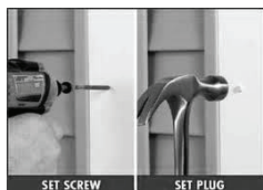
Cortex® Hidden Fastening System
