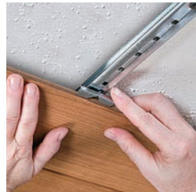
WoodHaven™ plank installation using Easy Up® tracks and clips
