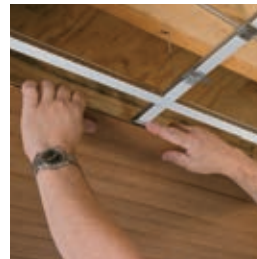
Position planks; slide and secure clips
