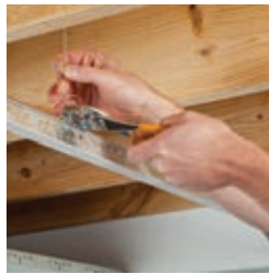
2 Suspend main beams with hanging hardware
