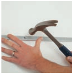
1 Install wall molding
