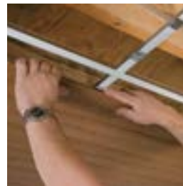
Position planks; slide and secure clips
