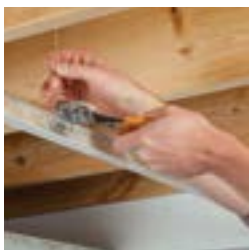
2 Suspend main beams with hanging hardware
