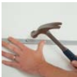
1 Install wall molding
