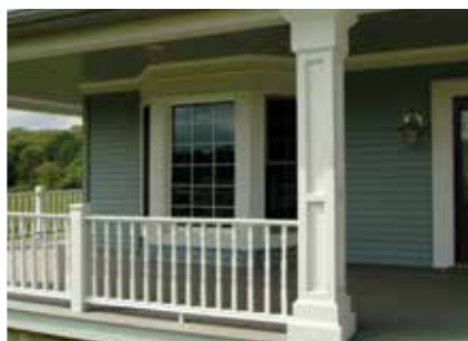
PORCH POSTS AND TRIM
