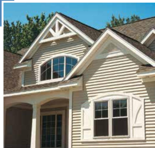
GABLES AND DECORATIVE SHUTTERS
